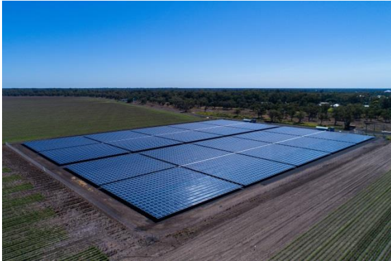
Caption: 4.77MWp Chillamurra Solar Plant at Goondiwindi Queensland, Australia
