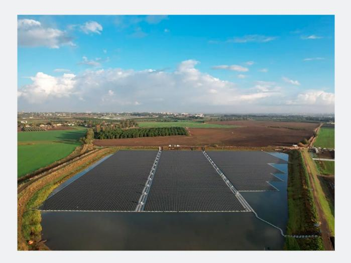
The biggest advantage of floating PV in contrast to conventional solar power plants is that no building land has to be acquired, leased or prepared for the power plant. In addition, the solar modules are inherently cooled by the water, so floating plants can have higher efficiency than those on land.
